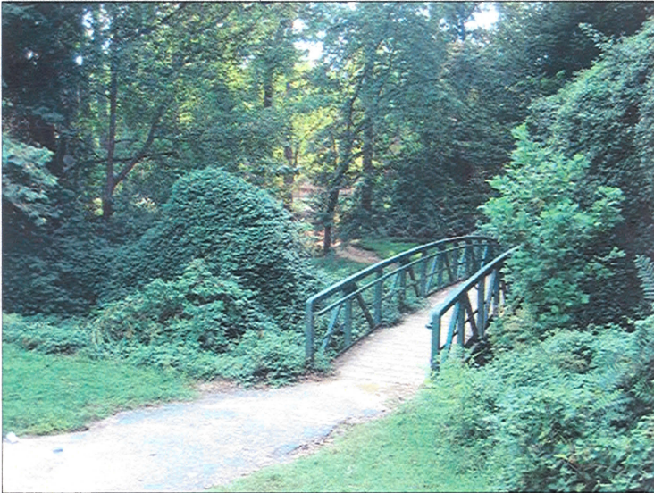
The existing Long Branch Bridge.
