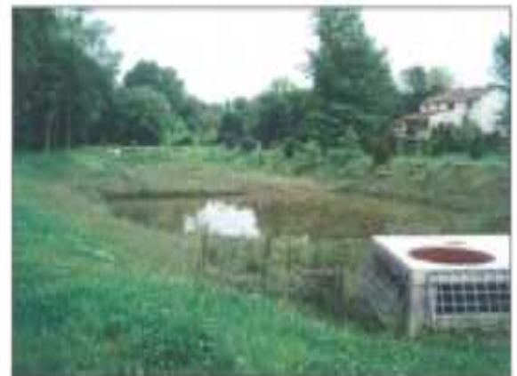
Figure 8. Piping Rock SWM Pond
