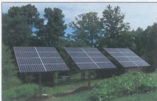
East Greenbush, NY Pole mounted 5.04kW system
