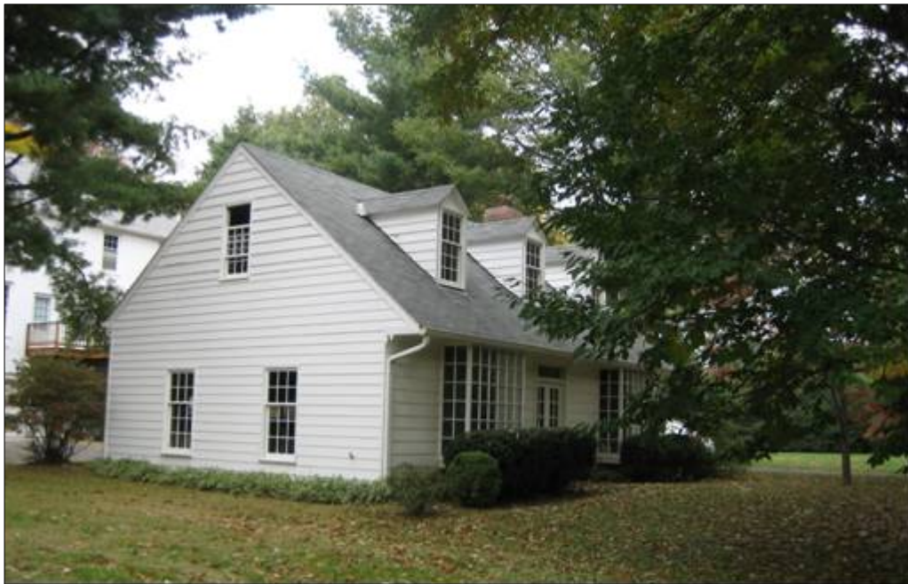
Figure 5 – the Garage / Workshop
