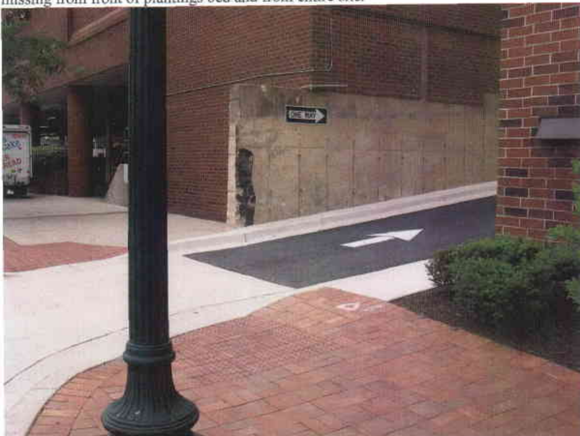
Brick paving not installed at crosswalk, sign missing.
