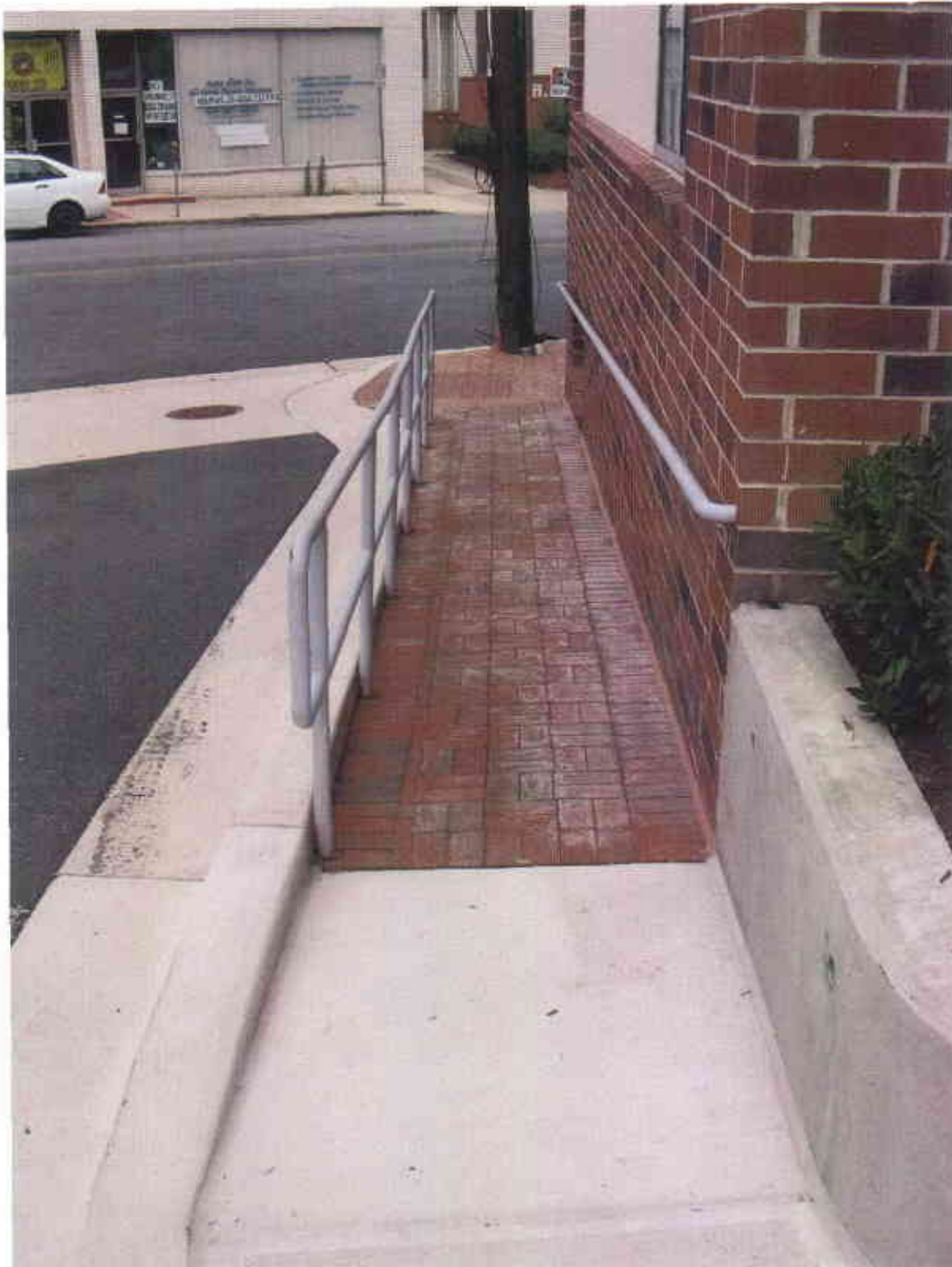
Internal walkways installed are narrower than the minimum 4' width required.
