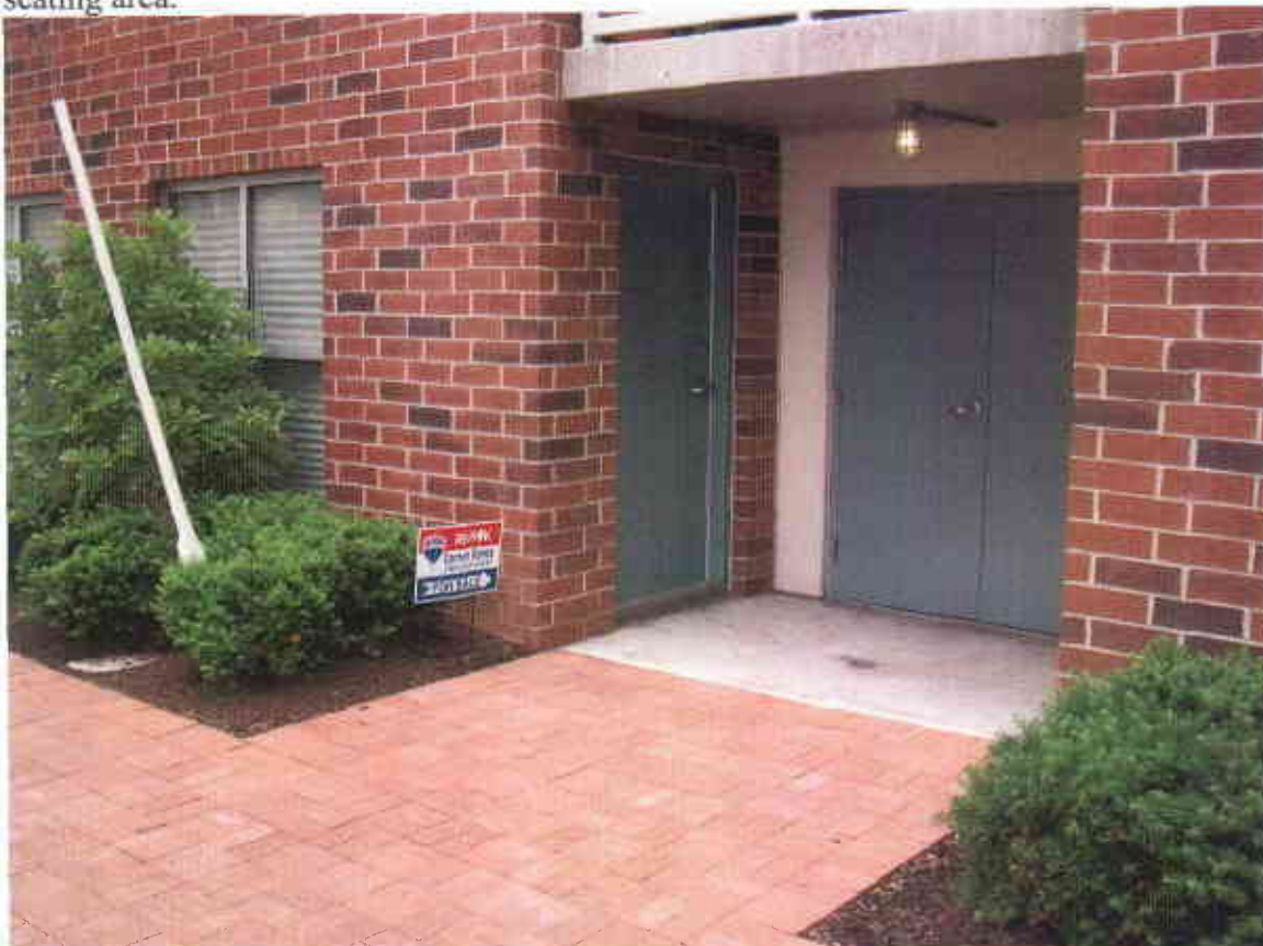
Granite paving has not been installed throughout site (required at entrances).
