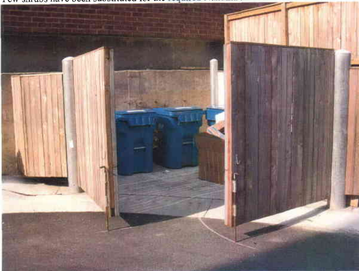
Dumpster not present, doors of enclosure do not open wide enough to accommodate required dumpster. Metal sleeve not installed.
