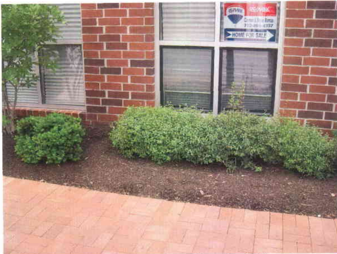
Only 1 of 2 required shrubs is present at left side of image. Candytuft groundcover missing from front of plantings bed and from entire site.
