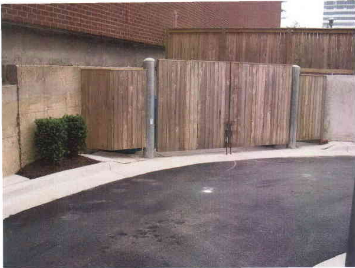
Yew shrubs have been substituted for the required Nandina shrubs.
