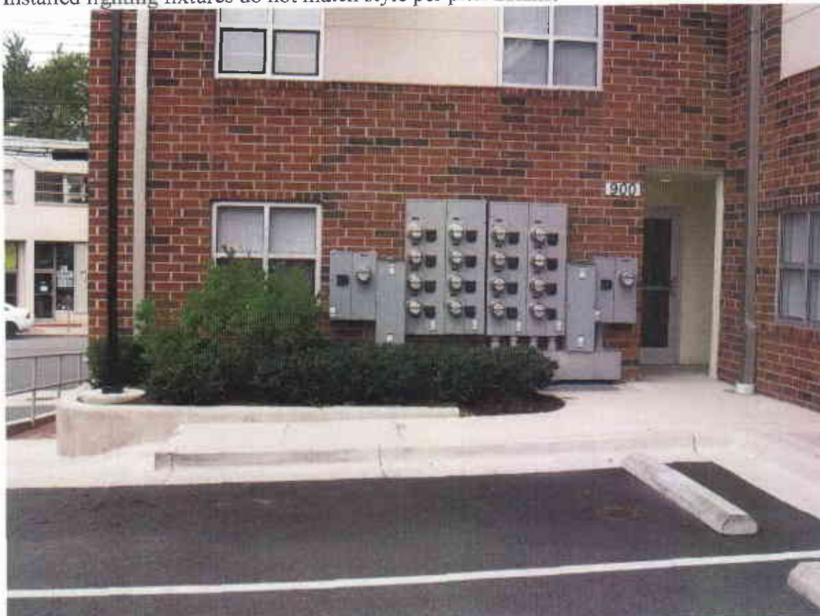
Magnolia tree missing from right side of landscape bed.
