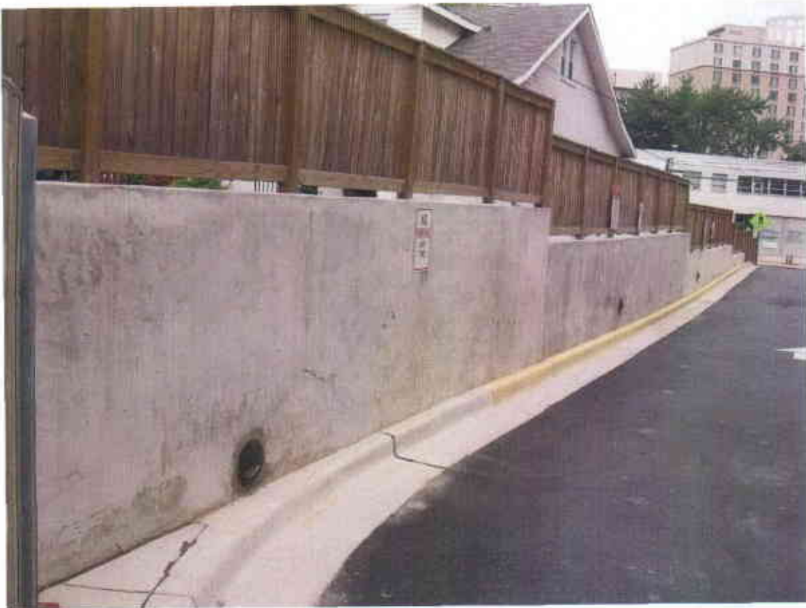
3 of the 4 required lights were installed within retaining wall.
