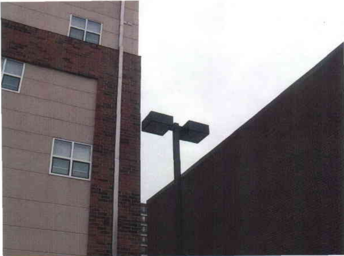
Installed lighting fixtures do not match style per plan details.
