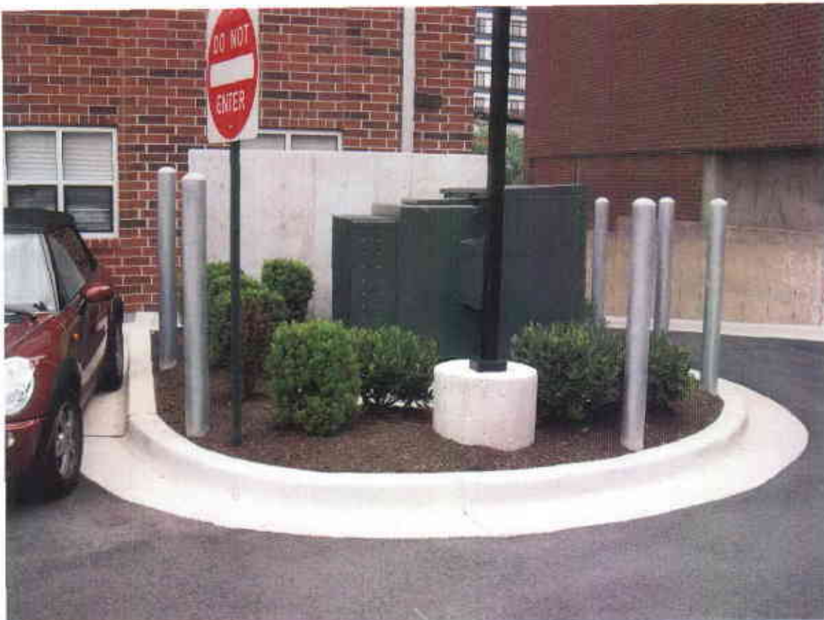
Large transformer box present; required tree absent from bed. Species and locations of landscape shrubs differ from approved plans.
