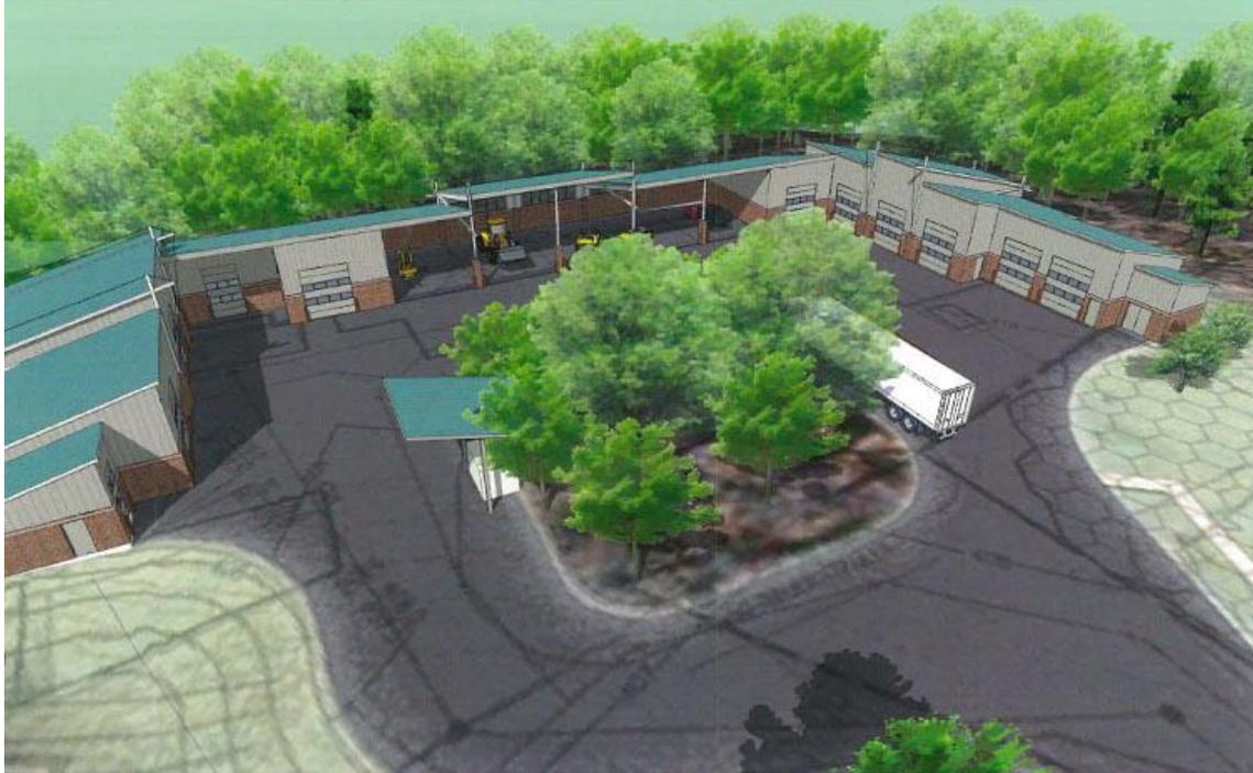
Because of the concern of durability, it was decided to pre-engineer the buildings steel structure and roof, but the first eight foot height of the walls would be masonry. Any walls above that level would be pre-engineered metal panels. The color of the metal and the ground-face masonry walls would match the materials of the Administration Building and tie all of the buildings on site together with a unified appearance. The Material Storage structures are treated in a like manner.
