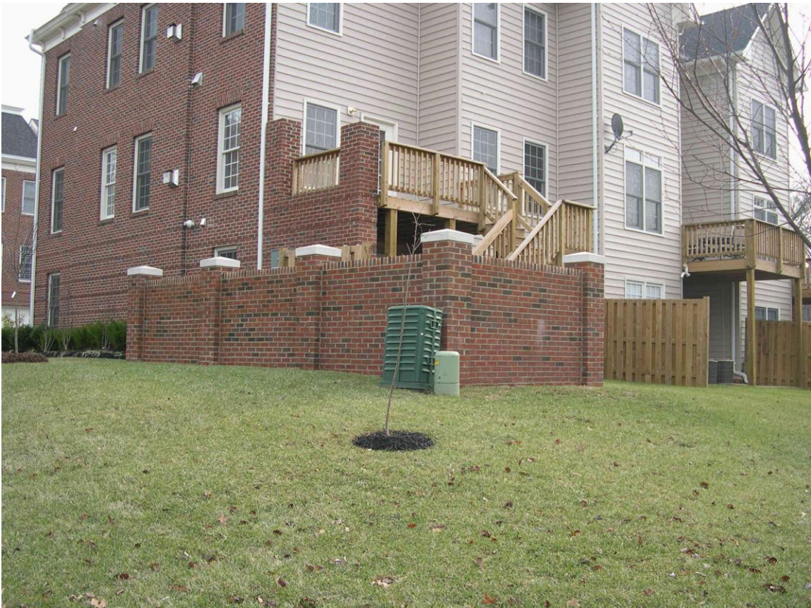
Masonry walls installed per plan, except wing wall (end sections) not installed per entrance feature detail.
