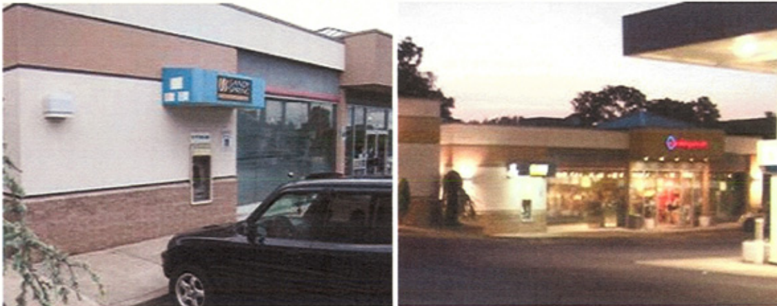
PHOTO 5: The canopy of the ATM machine is separate from the ATM dispensing machine. The ATM area is lit by the canopy and by adjacent two-directional wall fixtures.
