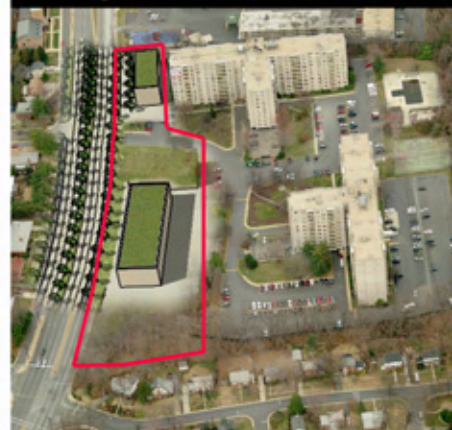
Development - Aerial View
