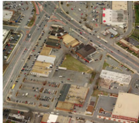
Existing - Site View
