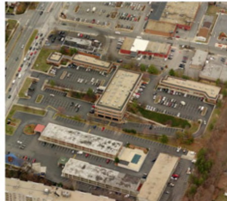
Existing - Site View
