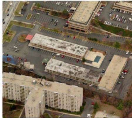
Existing - Site View
