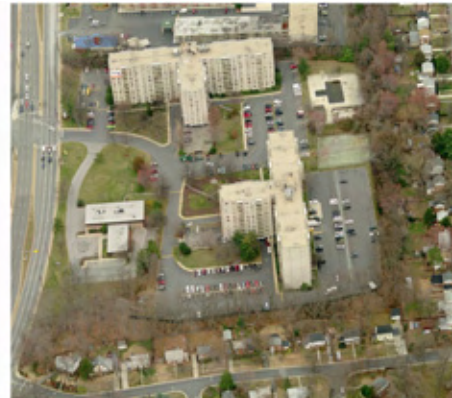
Existing - Site View
