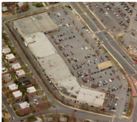
Existing - Site View
