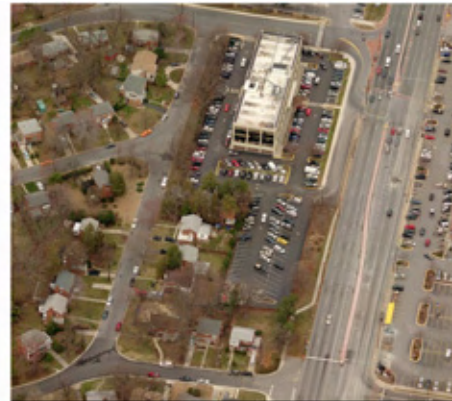
Existing - Site View
