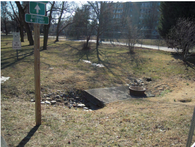
Erosion is occurring around two open throat inlets.
