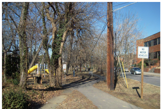
Above ground utilities that traverse the park detract from the park and should be placed below ground.
