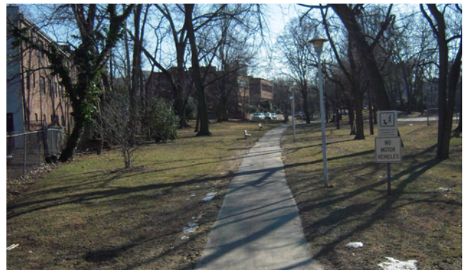
The primary path and bike trail is narrow and should be widened to accommodate pedestrians, cyclists, and service vehicles.
