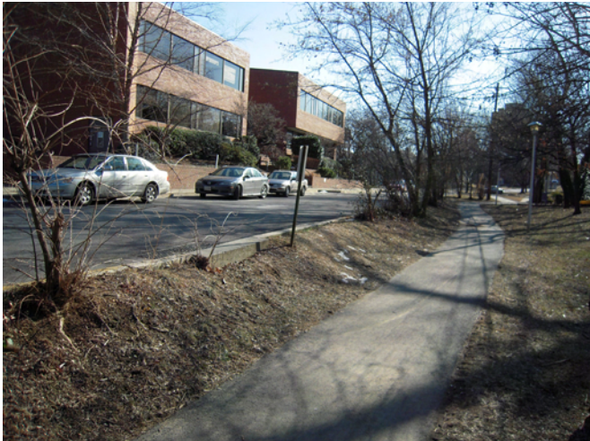
Grade change, erosion, and weedy trees along Glenbrook Road.
