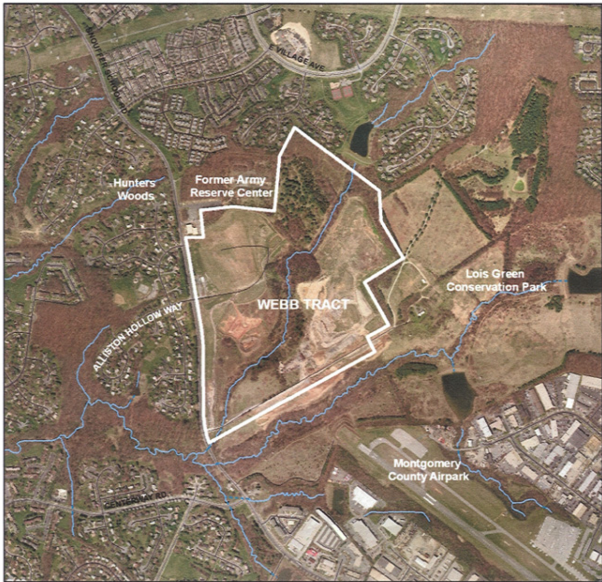
Figure 2: Aerial View of Webb Tract Property
