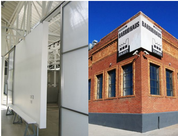
Multi-tenant Office, San Diego, CA Graham Downes Architecture
