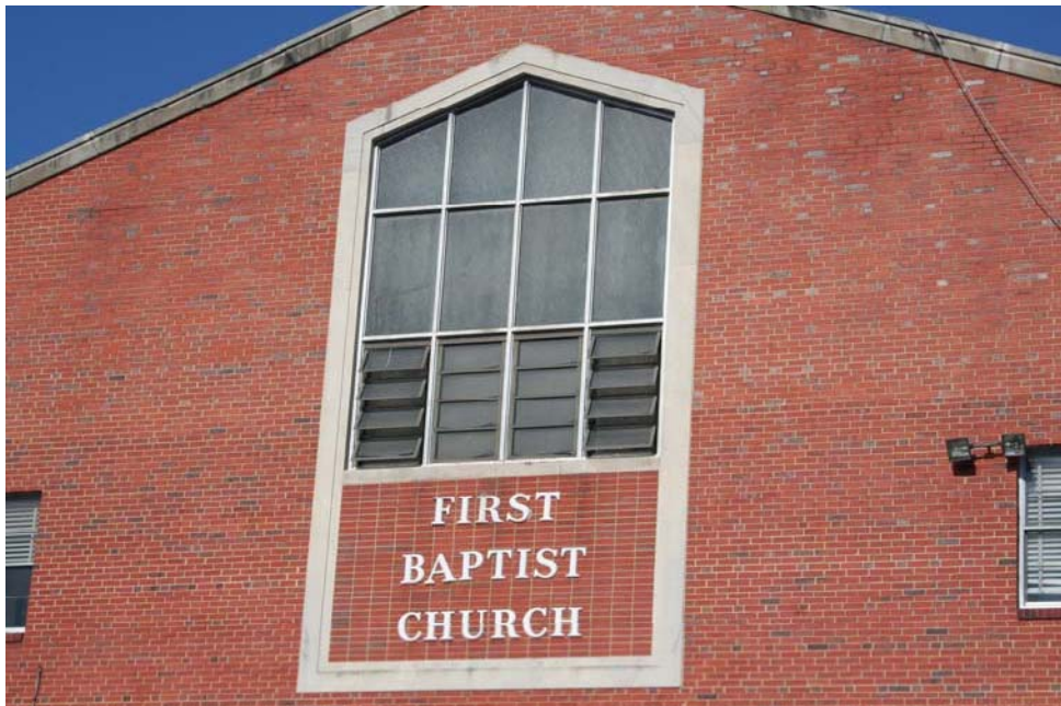
Silver Spring Baptist Church, south (rear) façade detail, Clare Lise Kelly, 02.19.10
