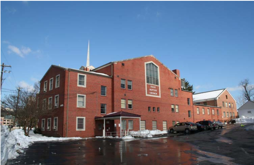
Silver Spring Baptist Church, south (rear) façade and partial west (side) façade, Clare Lise Kelly, 02.19.10
