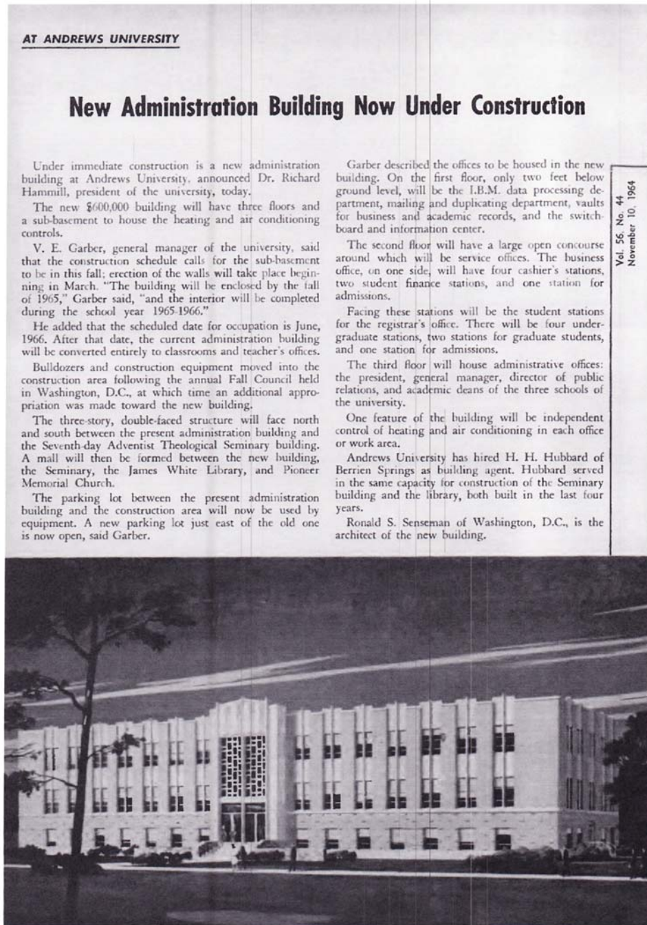
Andrews University Administration Building, Under Construction, 1964, Mich., The Lake Union Herald, Vol. 56, No. 44, 11/10/1964, p1.
