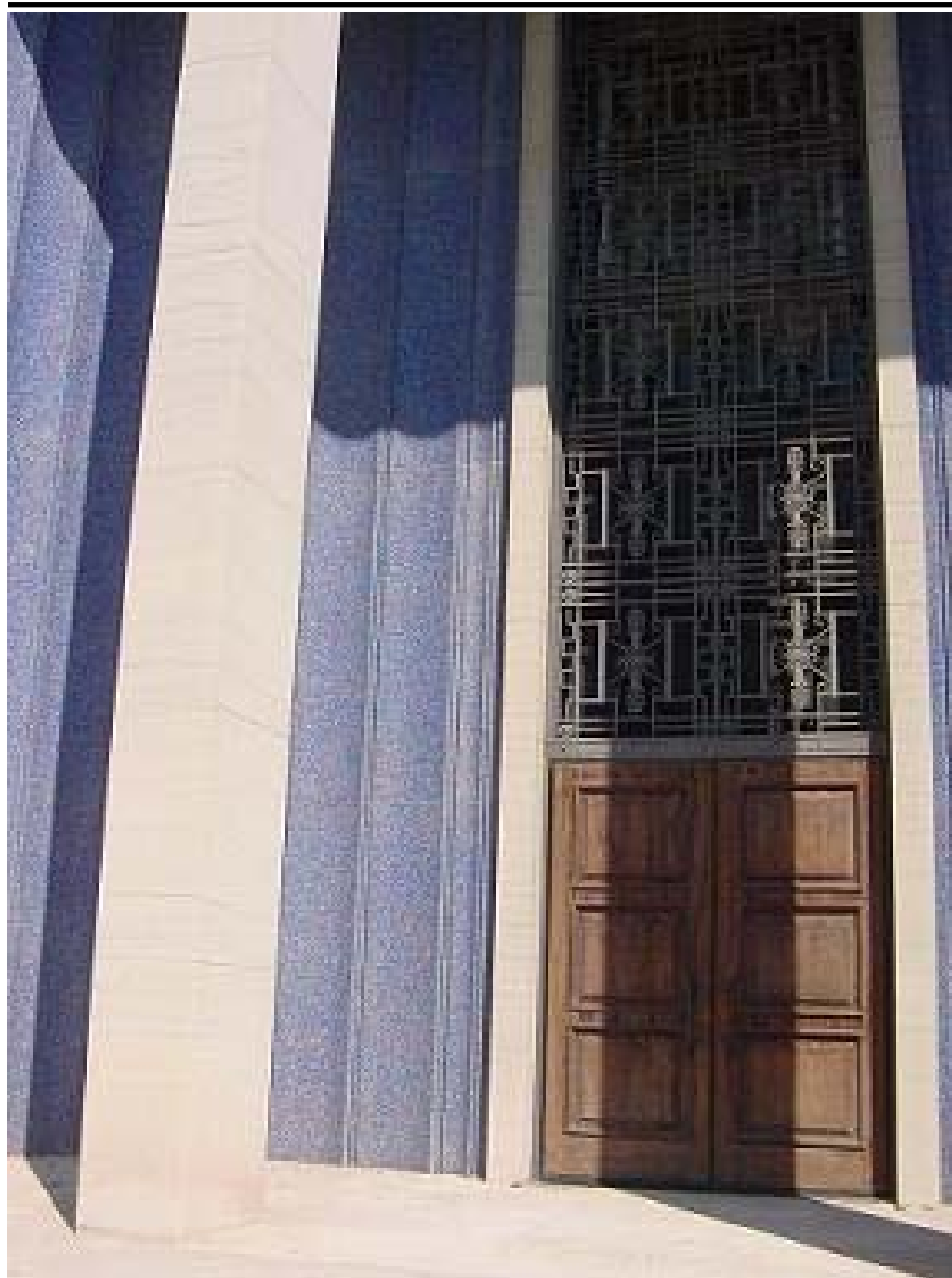
Senseman's 1954 Church of the Nazarene, Wash., D.C., now "The Mosaic Church." Front entryway details, including multi-colored tile, metal filigree work, wooden doors, limestone columns. SSHA Photo
