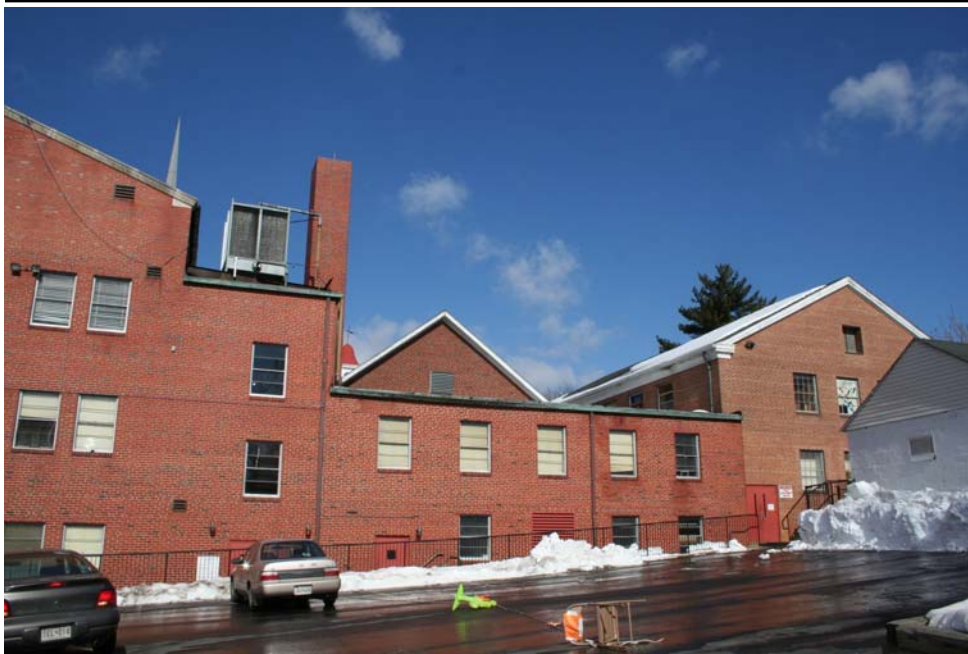
Silver Spring Baptist Church, partial south (rear) façade, Clare Lise Kelly, 02.19.10
