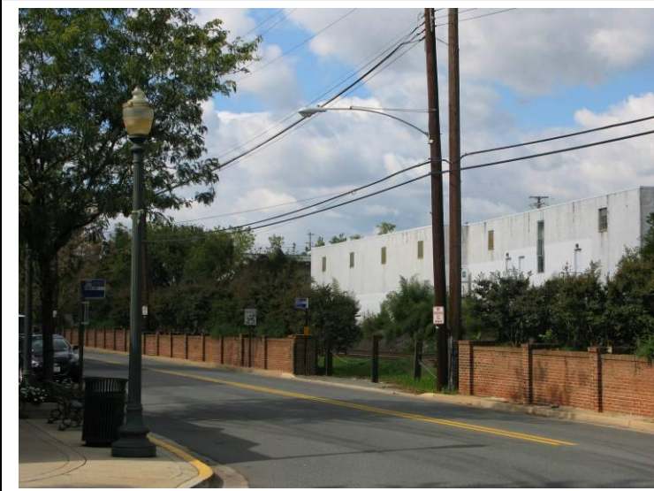
The back façade of existing development along Metropolitan Avenue is highly visible from Antique Row.
