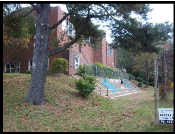
Figure 3 South side of the building from Forest Glen Rd
