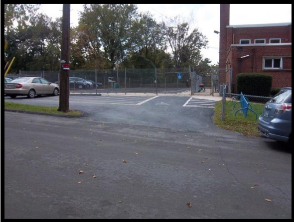
Figure 6 Pool area (to be removed and replaced with 20,000 SF addition)
