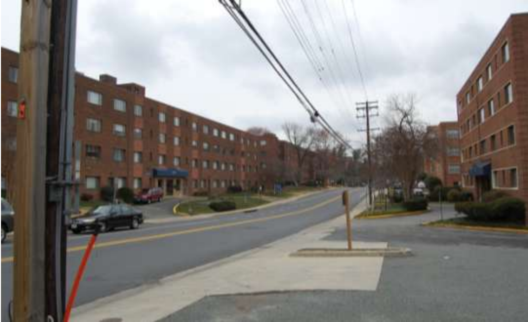
Views west along Battery Lane from 4857 Battery Lane
