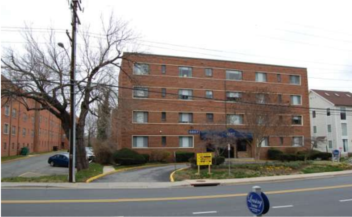
4857 Battery Lane "Glenwood At Battery Lane"-Site 1 Proposed Site for Building "A"
