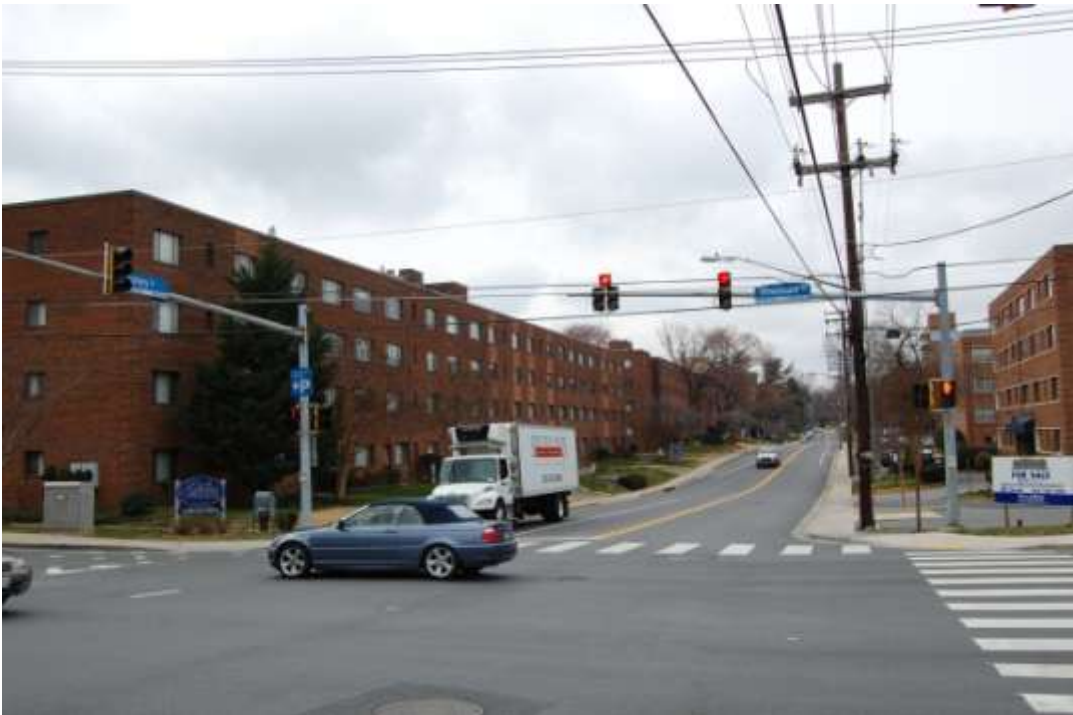
Views along Battery Lane looking west-Sites 2 and 3
