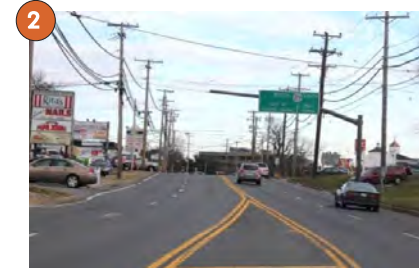
2 Lack of sidewalks
