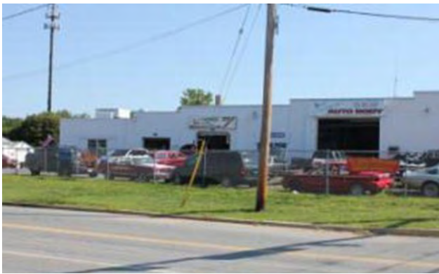
Examples of Existing Facades: Unimproved facades along Main Street MD 198
