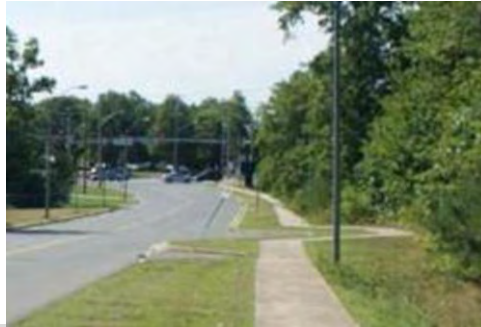
Examples: Existing retail access road at MD 198
