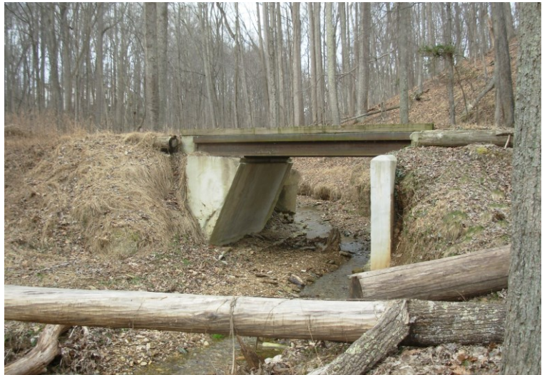
Potter Property: bridge crossing, April 2010
