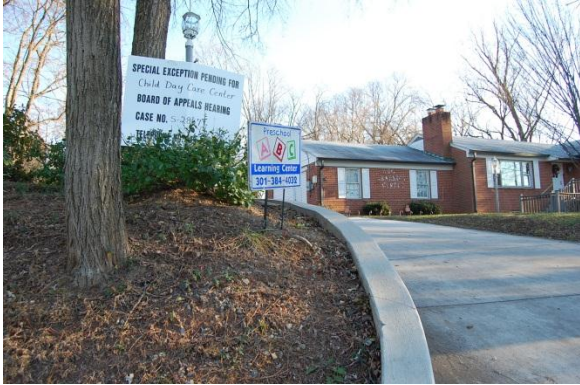
Figure 1: Front of Structure
