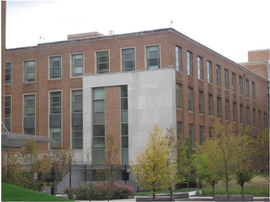
Southeast façade with limestone panels where connector wing once stood, 2011
