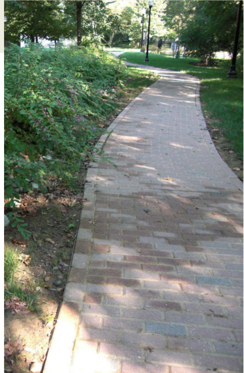
Existing buffer park walkway
