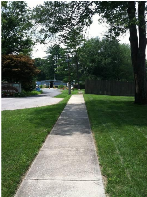
Image 1: Existing Sidewalks North Side Landgreen Street, View West
