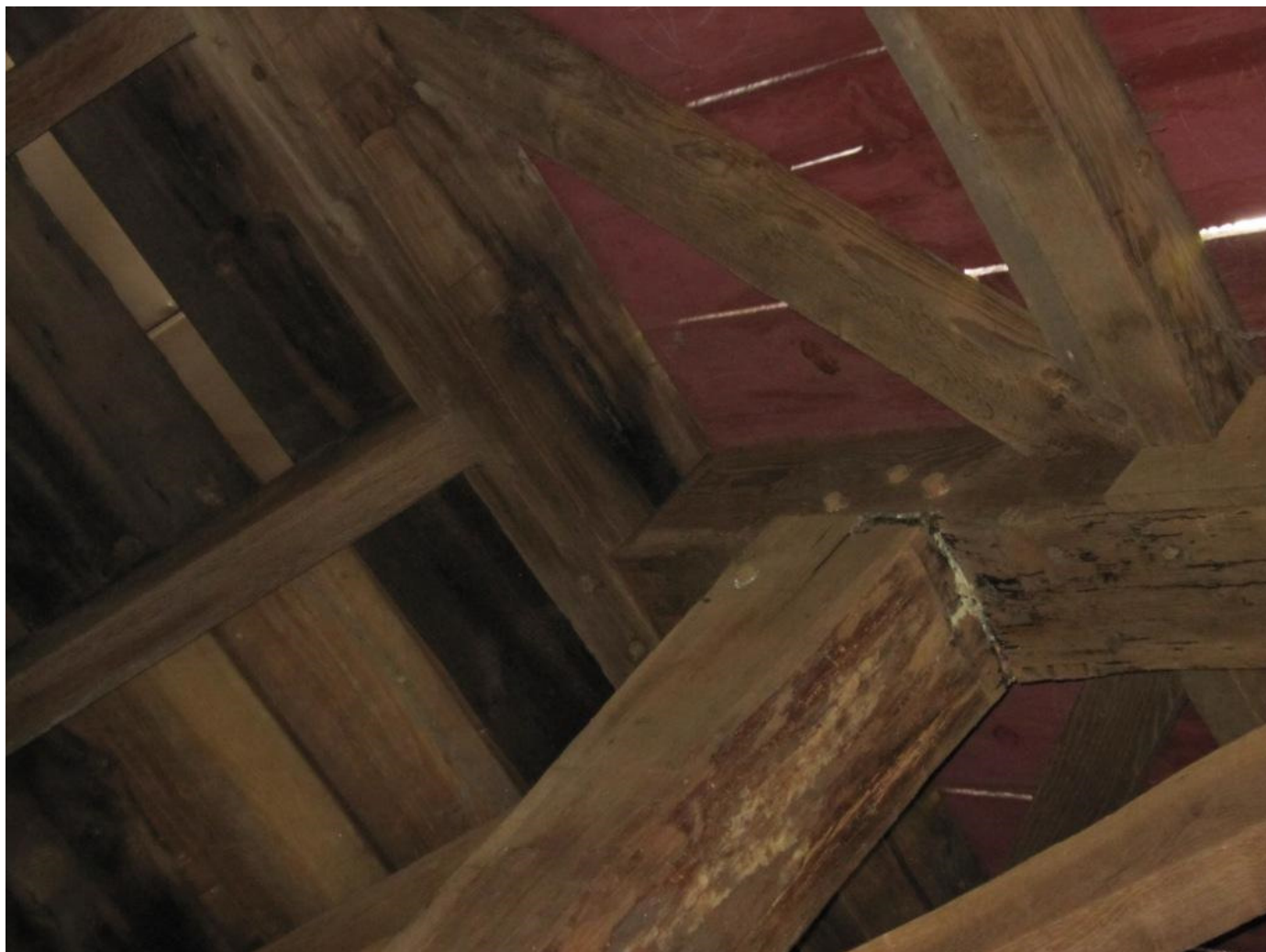
Figure 19. Framing system shows pegs and diagonal braces.
