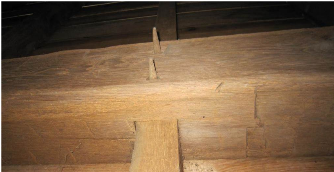
Figure 20. Pointed Pegs between Post and Tie Beam.
