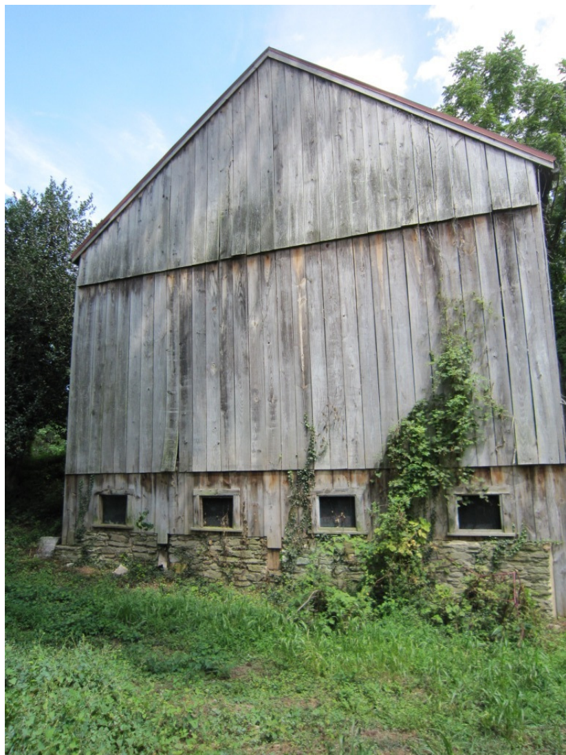
Figure 17. View of Southwest gable end.
