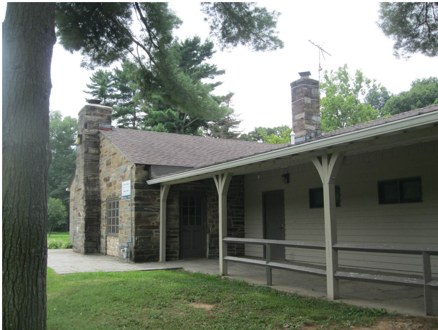
Figure 18. View of Meadowbrook Recreation Building, northwest corner.
