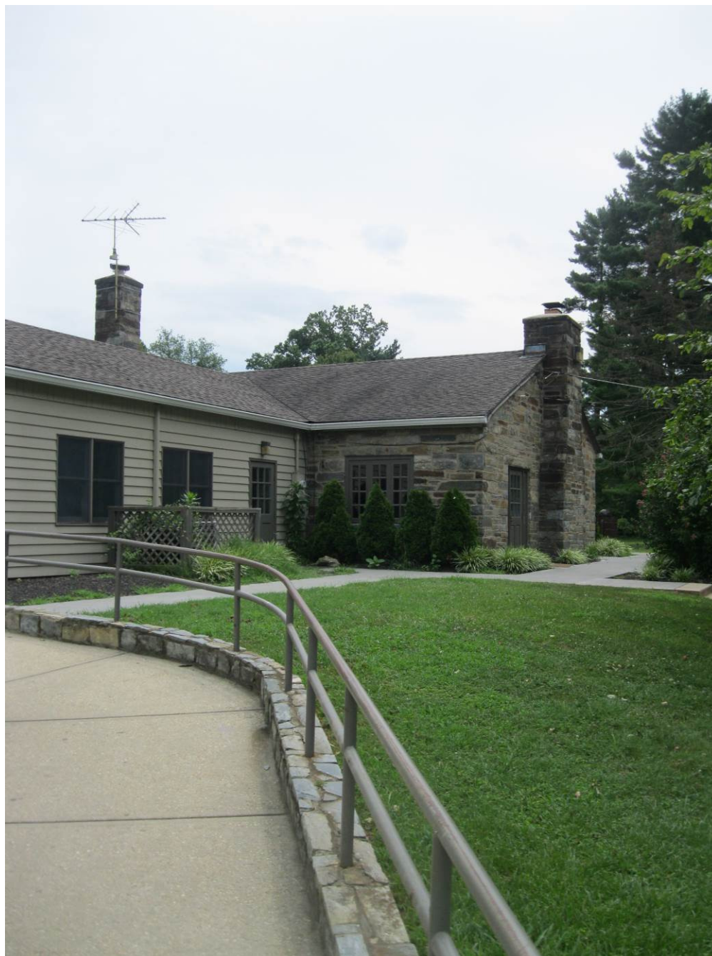
Figure 20. View of Meadowbrook Recreation Building, northeast corner.
