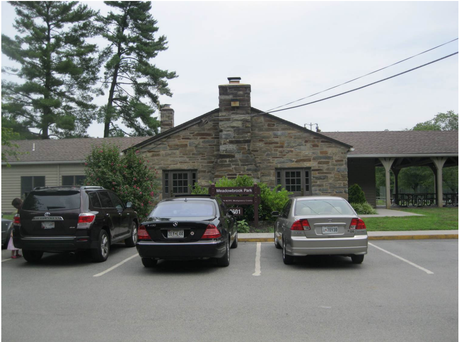
Figure 14. View of Meadowbrook Recreation Building, east (front) façade.
