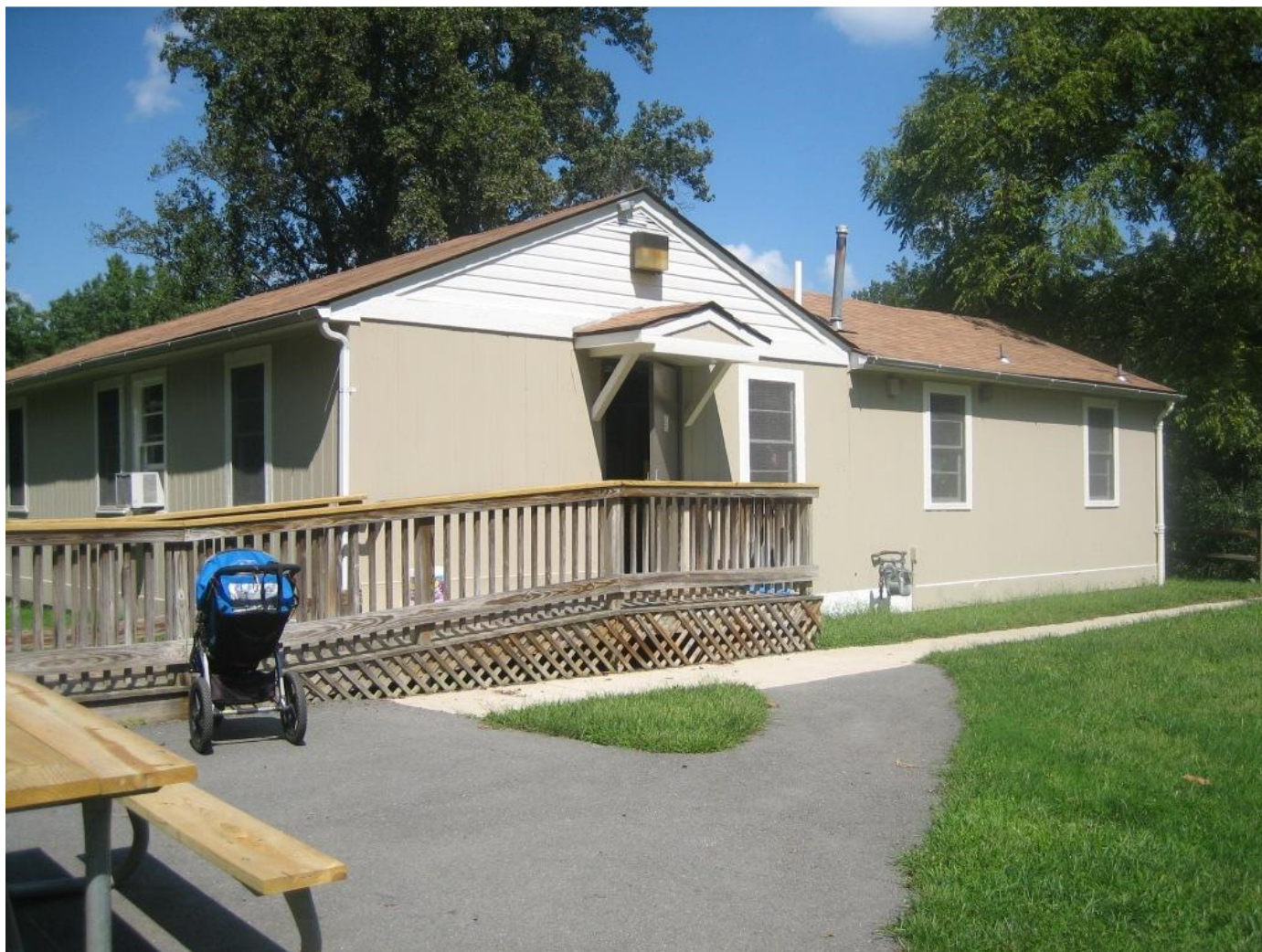
Figure 12. View of Ken-Gar – Palisades Recreation Center, west and south (rear) elevations.
