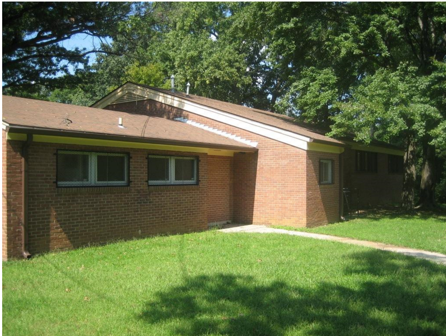
Figure 11. View of Veirs Mill Recreation Building, east (rear) elevation.
