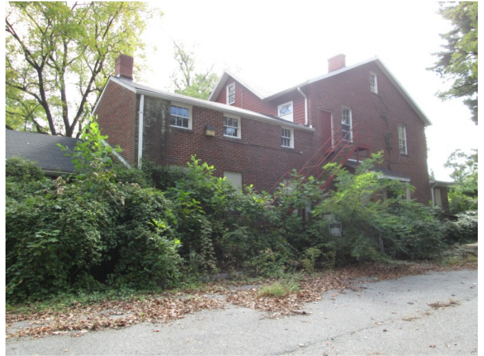
West side view showing main 1850 house, 1860 addition and 1950s garage.
