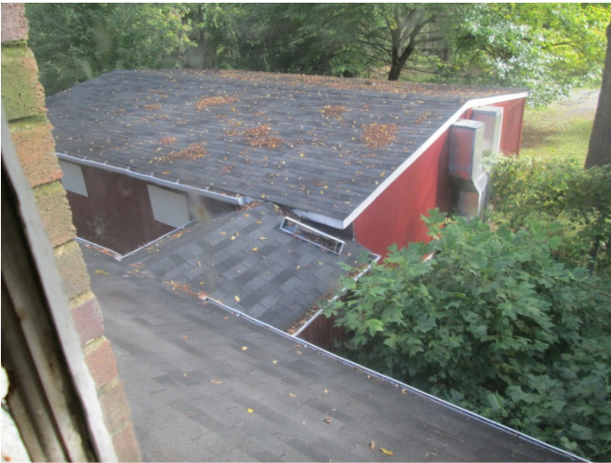
View from 2 nd floor of 1860 addition showing roof of enclosed side porch, roof of passage to trailer and trailer.
