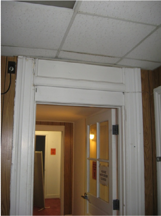
Original doorway into addition
