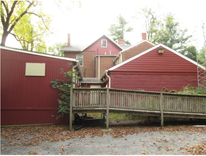
Rear view with garage on right and trailer on left, Handicap ramp in foreground with the passageway to Trailer behind it.
