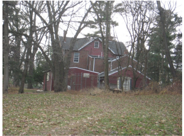
Stubs House rear, north façade
