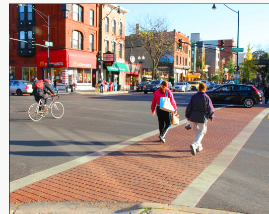
Brick crosswalks demarcate pedestrian areas within the intersection
