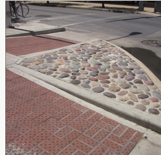
Special paving in handicap ramps provide visual and tactile cues to handicapped pedestrians
