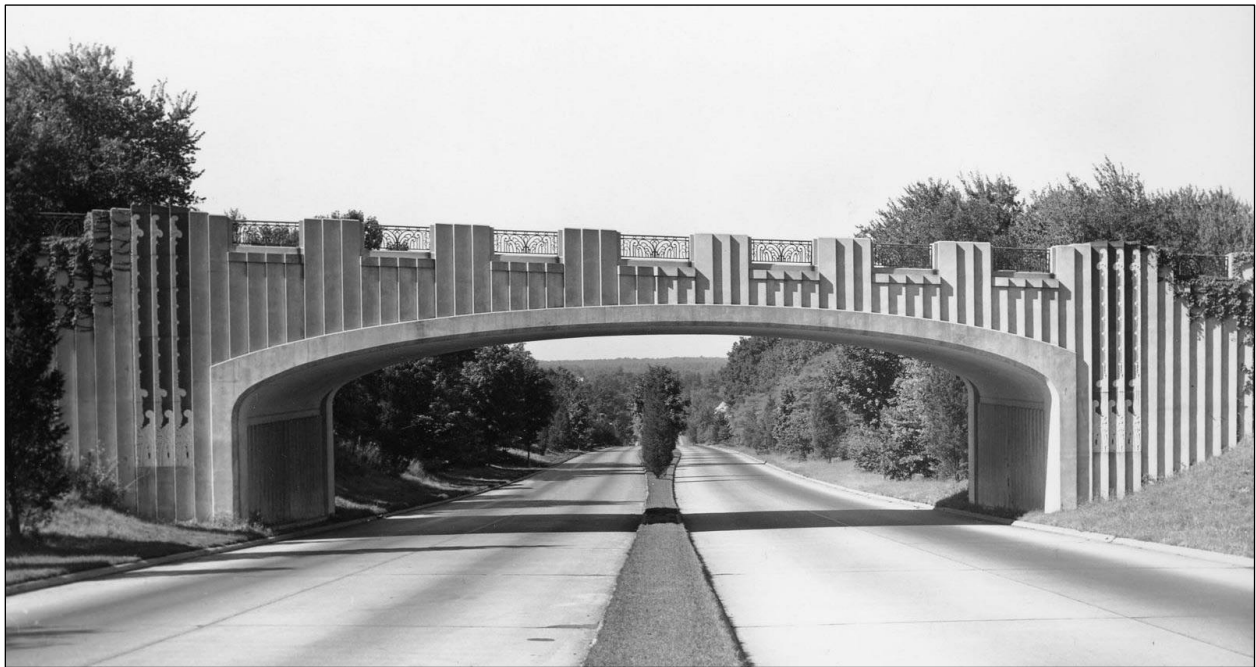
Figure 1-18: Example of a Shallow Arch Structure Bridge
