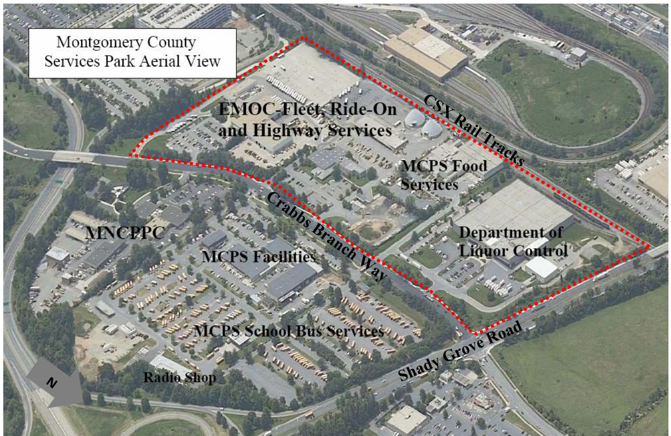
Overview of the Montgomery County Service Park, looking southwest
