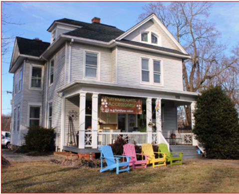
Adaptive reuse of the former 1903 Holly Cottage as a commercial building
