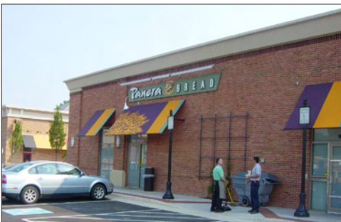
Lansdowne, VA: The rear facade of the building has a secondary entrance that is articulated similarly to the front facade.
