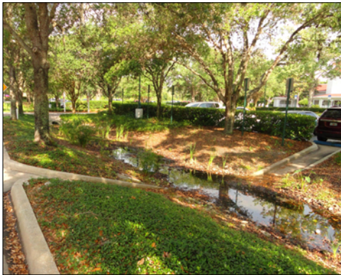
Orlando, FL: Landscaped islands in a parking lot provides an area for stormwater collection.
