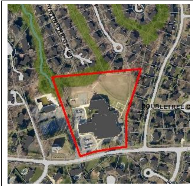
Aerial photograph showing surrounding residential pattern and proximity to Watts Branch Stream Valley
