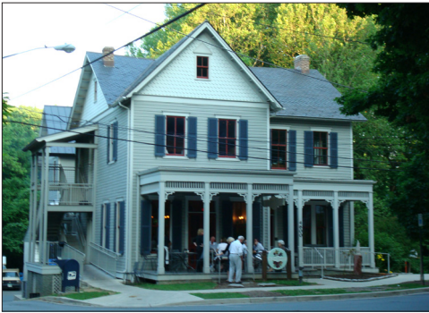
Garrett Park, MD: Adaptive reuse of an existing building into a retail use.
