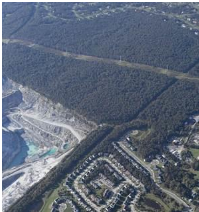
Serpentine Barrens Conservation Park with the County's largest quarry and residential development in the foreground and background
