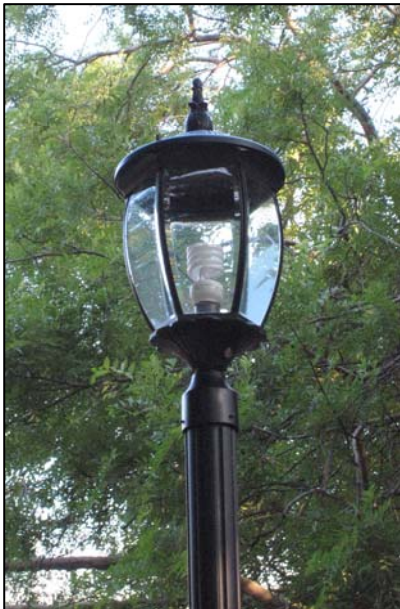
Image 5: Post top fixture at Caroline Freeland Park
