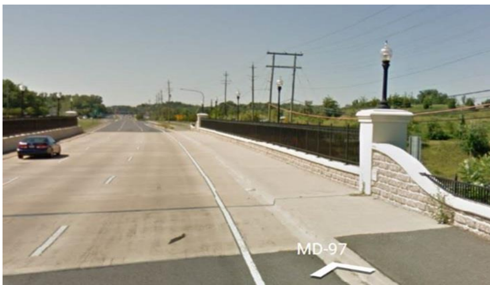
Figure 11 - Pedestrian Light Fixtures on Columns and Stamped Concrete
