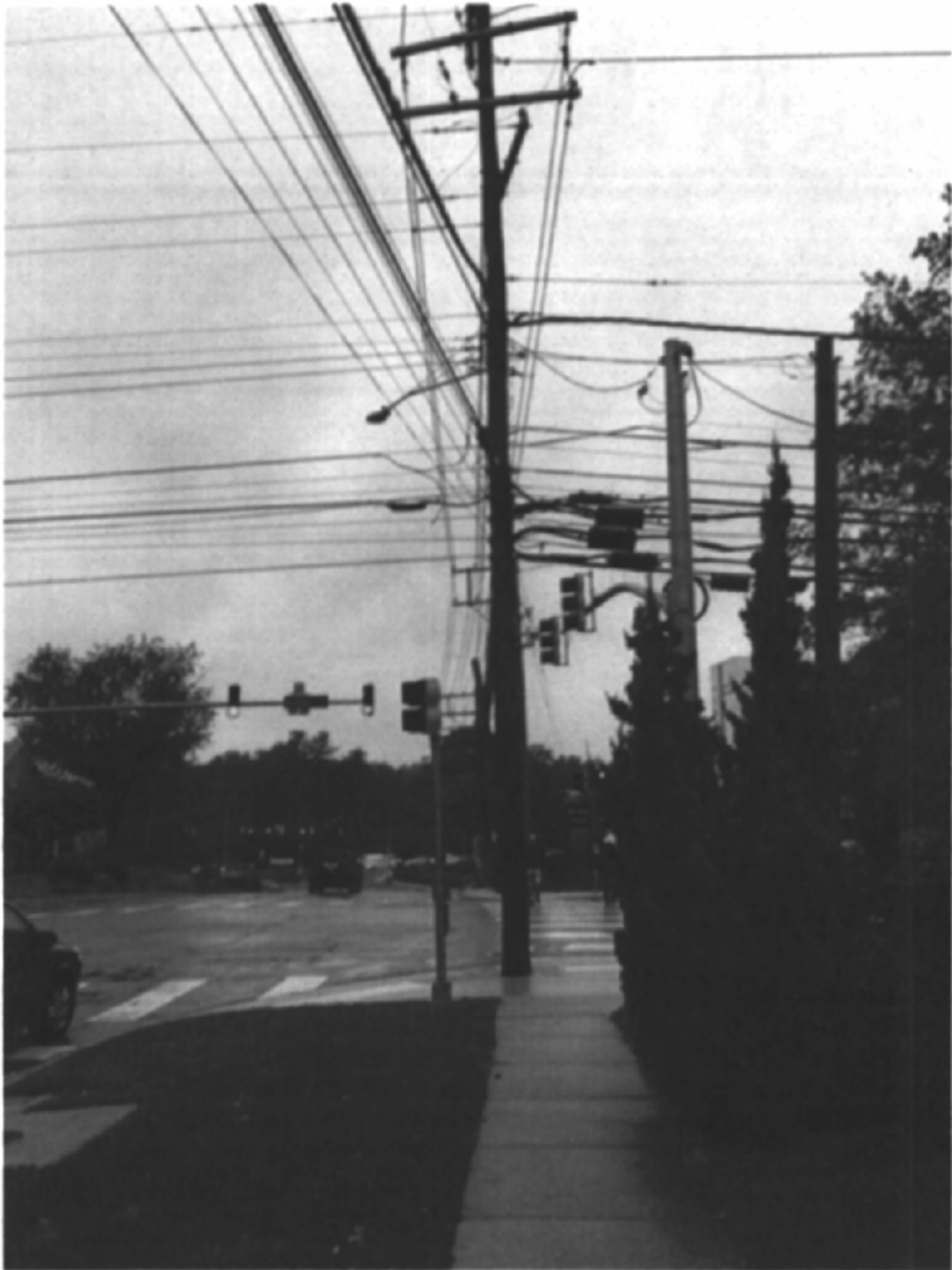
Utility lines and poles at the corner of Westbard Ave. & Ridgefield Road.
