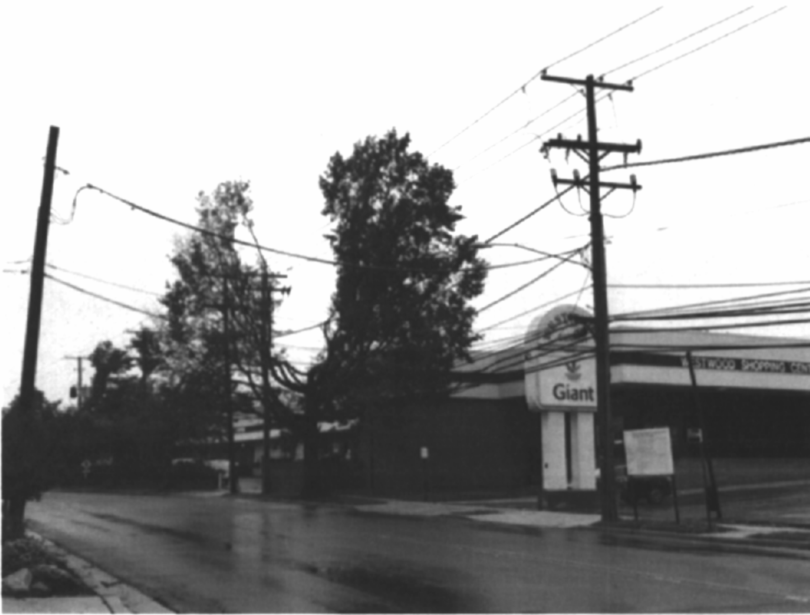
Westbard Avenue utility poles and lines by Westwood I.
