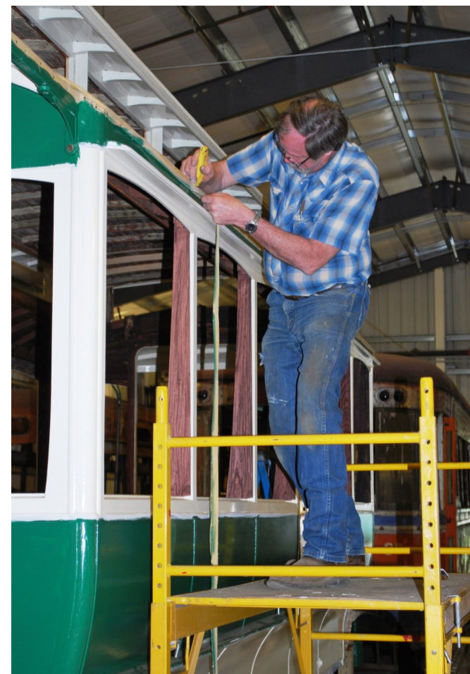
Upon his return on May 7 th , Keith Bray trims the excess canvas to prepare for painting the roof on CTCO 522.
