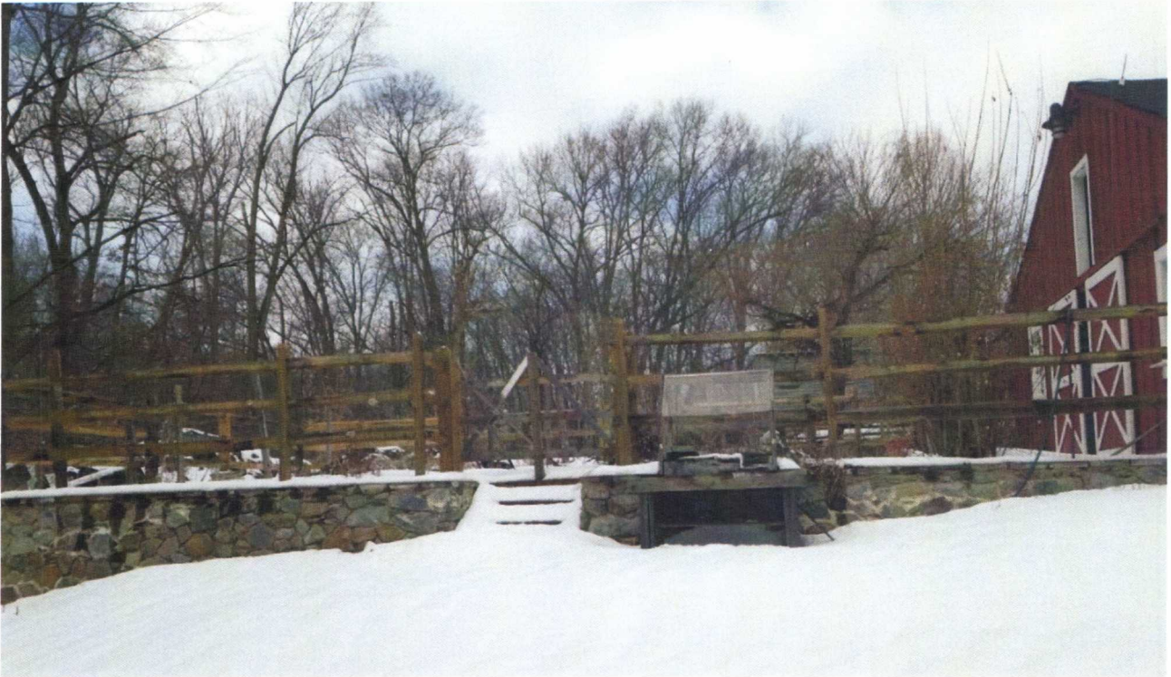
Figure 2 - Stone Wall Terrace and Fence in rear Conservation Easement area of Lot 175
