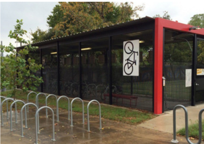
Bicycle Parking at the Kramer Station in Austin, Texas
