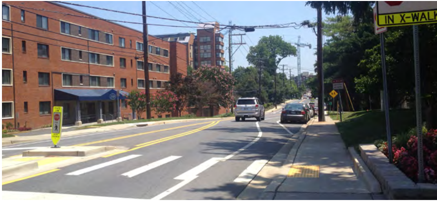
View of Battery Lane looking east
