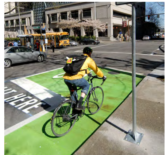
Intersection improvement with bike boxes Source: City of Portland
