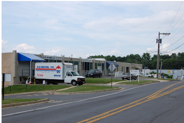
Industrial/hybrid retail with customer sales in front and production in back
