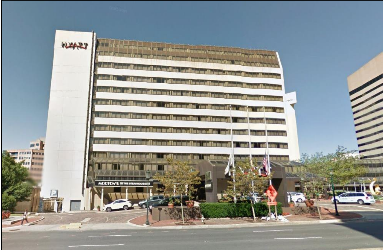
Figure 3 - Existing Site, View from Wisconsin Avenue
