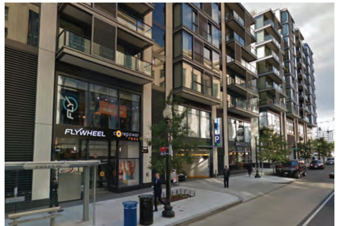
This parking entrance is designed to blend with the ground floor retail design, and has a limited driveway width to reduce interruption along the sidewalk. Source: Google Street View
