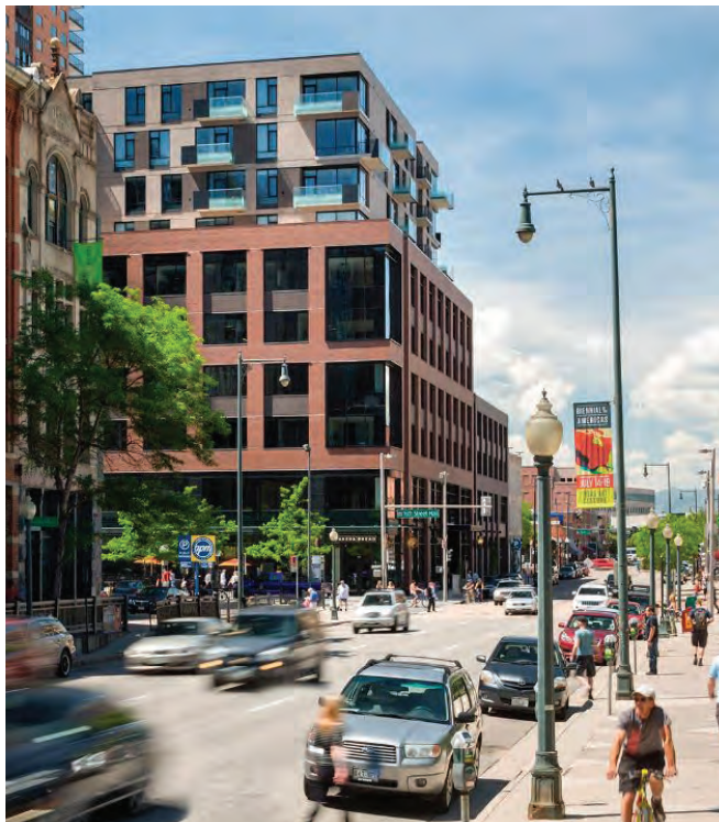
This mixed-use building combines commercial lower floors and residential upper floors, which are stepped back. Source: Gensler
