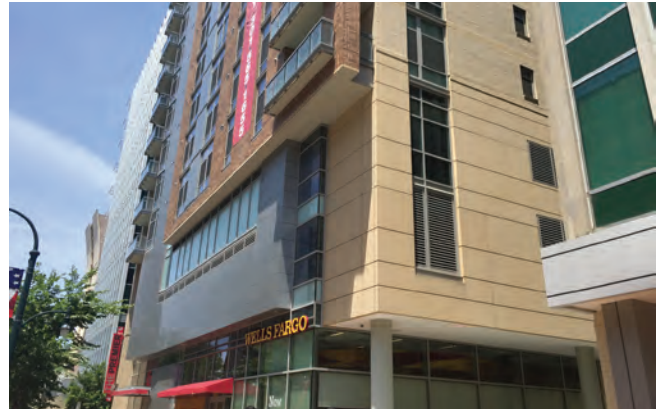
Structured parking floors are screened with a facade treatment consistent with the design of the building.
