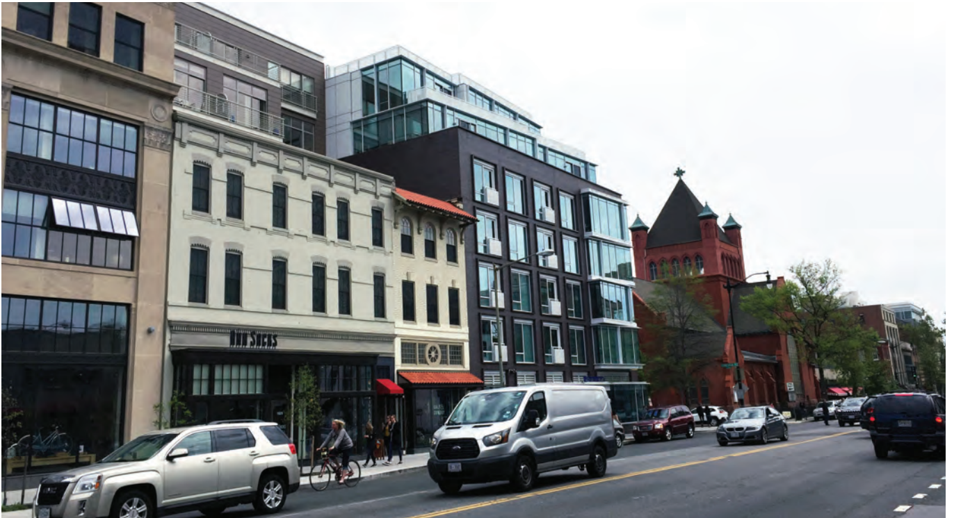
Buildings along 14th Street NW in DC step back from the street above a low to mid-rise base to maintain the main street character and scale.
