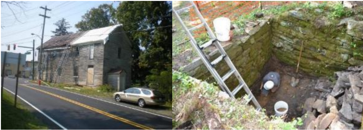
Left: Darby Store, prior to rehabilitation and move. Right: Thomas Mill, in need of stabilization or reconstruction.
