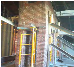
Chimney earthquake damage
