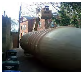
Underground tank for sprinkler
