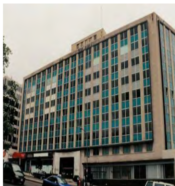
Existing Facade on Connecticut Avenue
