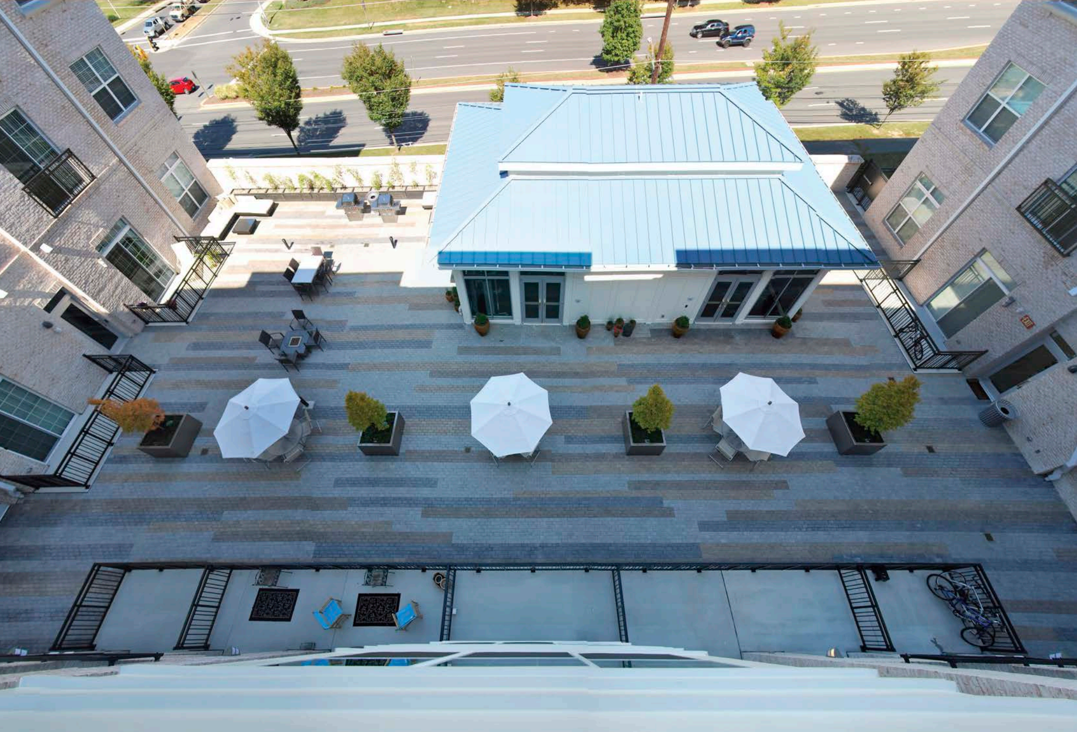
PARAMOUNT EAST ROOFTOP TERRACE Gaithersburg, Maryland
