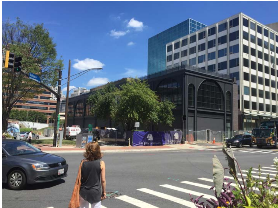
Figure 2: Looking toward Reed Street right-of-way from Bethesda Avenue (looking north)
