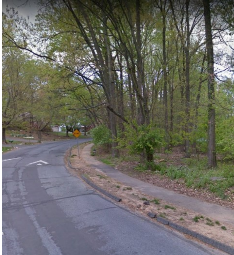
Figure 4: Marcliff Road sidewalk
