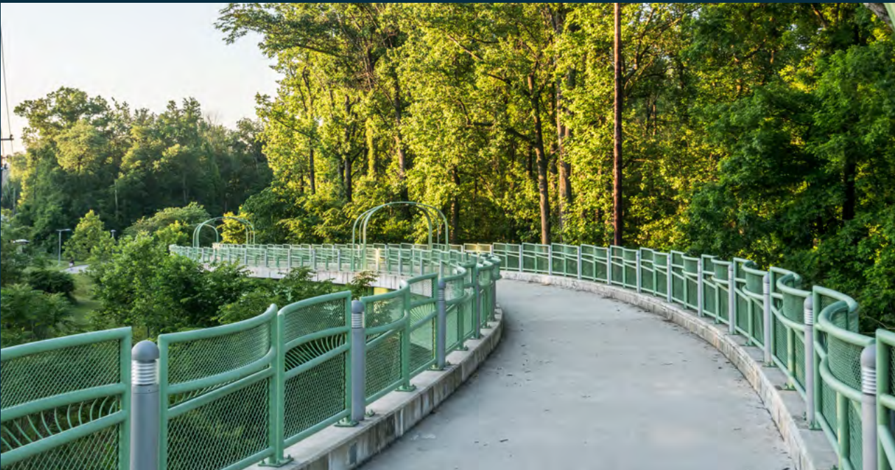
Rock Creek Trail Bridge
