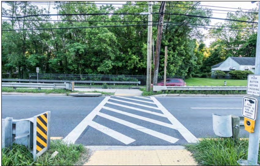
Existing Matthew Henson Trail crossing
