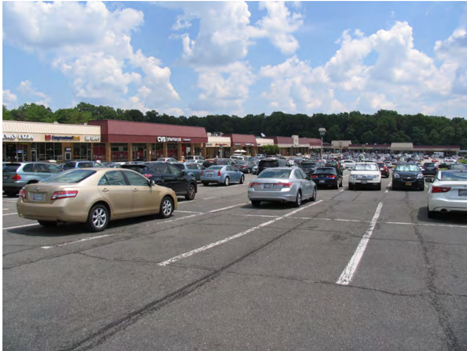
1. Overview of Cabin John Shopping Center, Facing West
