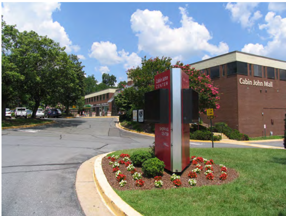
2. Overview of the Cabin John Mall, Facing Northeast
