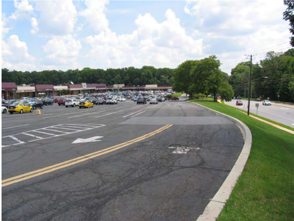
5. View Southeast from Southwest Corner of Cabin John Shopping Center Property, Along Berm Separating Shopping Center Driveway from Public Way on Seven Locks Road (right of frame)
